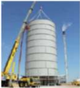
FLARE INSTALLATION Modular design simplifies the installation of our ground flares.
